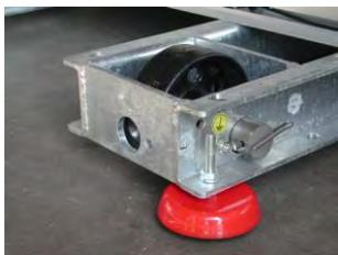
Subsequently is illustrated how assembly the vibration dampers on transformer. Fig. 4
